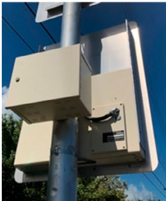
Most common LED Signage Installation
